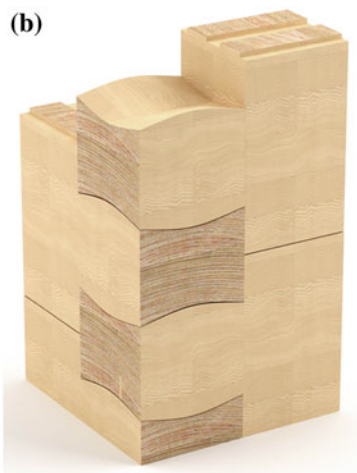
Fig. 3.18 Types of connections in log construction; (a) the old type, (b) the new type
