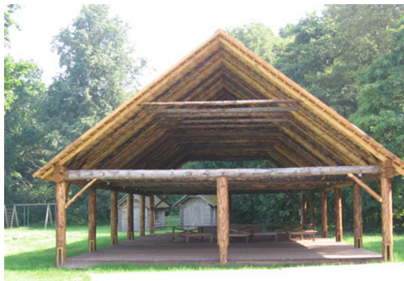
Fig. 3.29 Post and beam structural system
