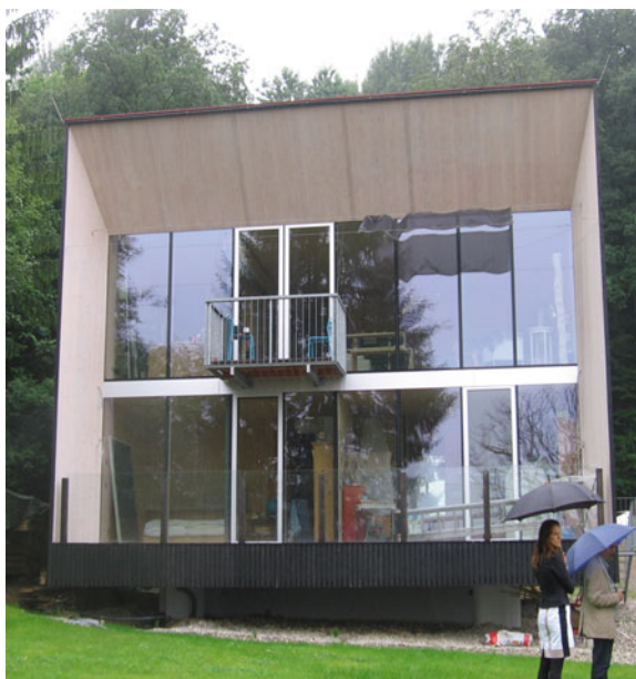
Fig. 4.30 Two-storey single-family house with HGV wall elements, built in Eichgraben (Austria)
