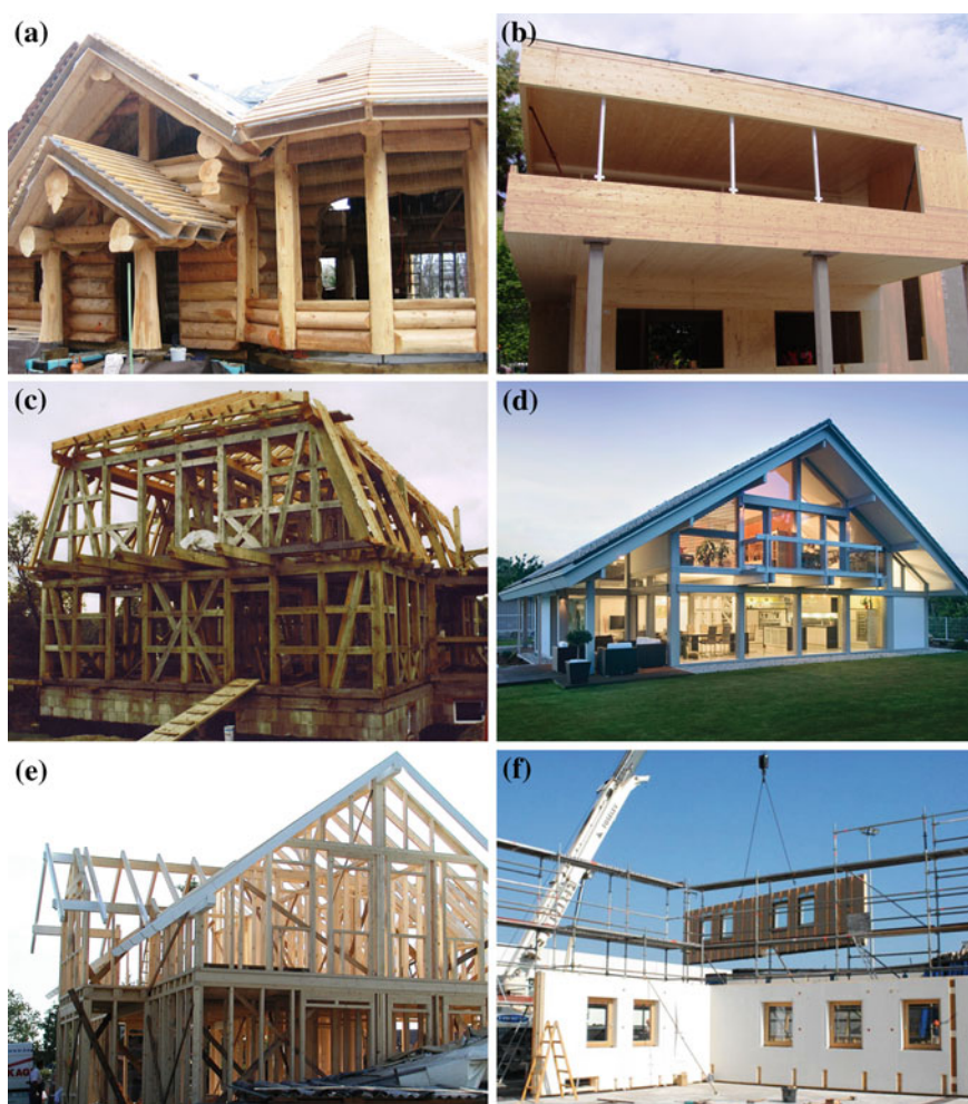
Fig. 3.15 Overview of the basic structural systems in timber construction; (a) log construction, (b) solid timber construction, (c) timber-frame construction, (d) frame construction, (e) platform-frame construction, (f) panel construction; photograph by F. Kager
