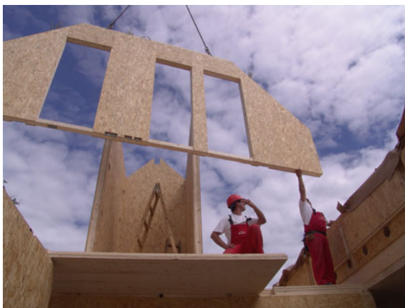
Fig. 3.19 Platform-type erection in the massive panel timber construction, photograph by F. Kager
