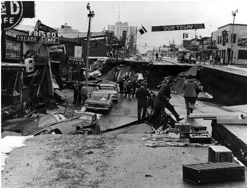
Figure 4-1 Roadway and buildings damaged in an earthquake
